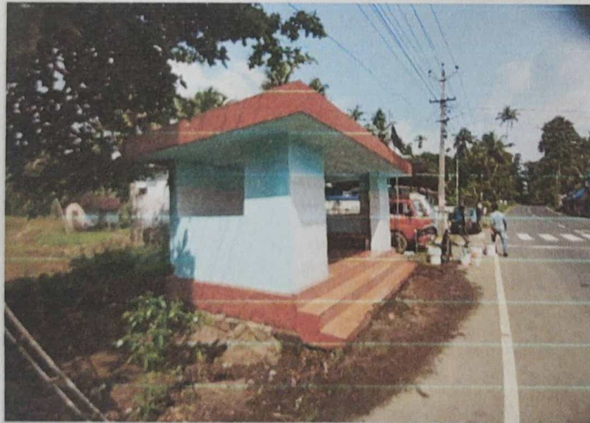
Photo 12.2 : Mutholapurom bus waiting shed after painting.
