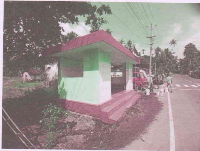
Photo 3.2 : Mutholapurom bus waiting shed after painting.
