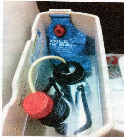
Flush Tank Bank
